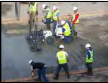
Expo – Concrete Placement
