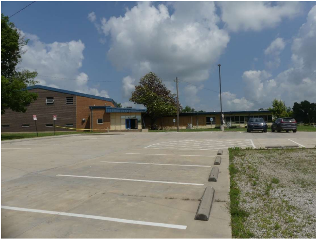
1. Front, south side, of the school.
