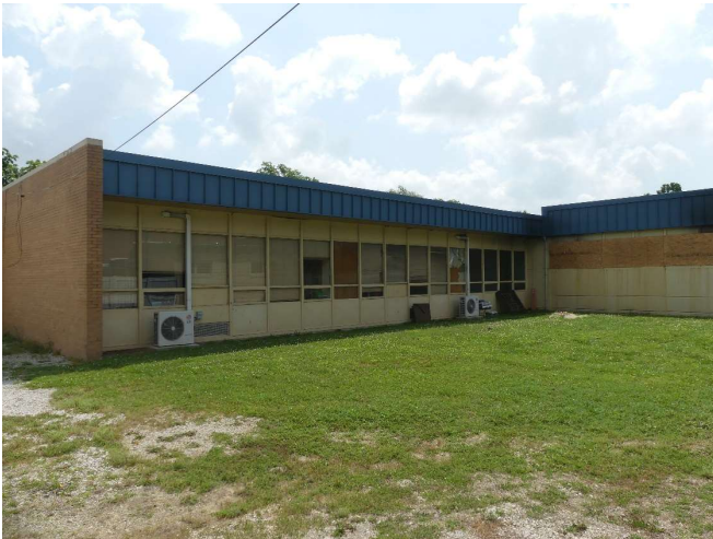
7. West side of the east building section.
