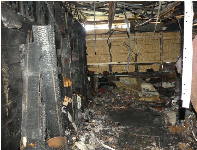
23. View into the kitchen area in the east-west oriented building segment.
