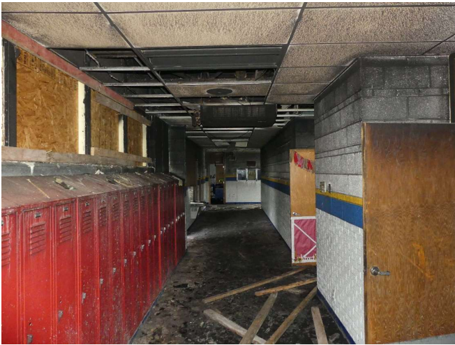
15. Looking east along the east-west hallway.
