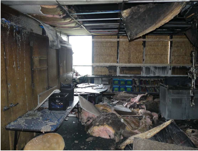
21. View into the west classroom in the east-west oriented building segment.
