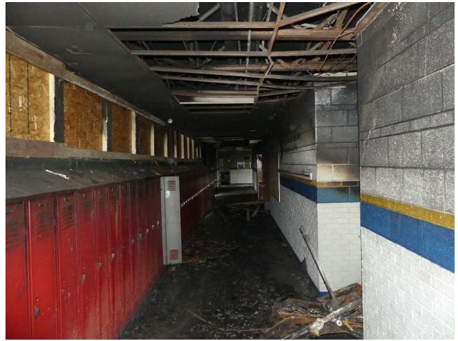
14. Looking east along the east-west hallway.
