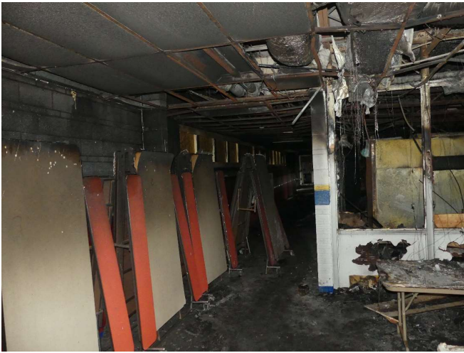
13. Looking east into the east-west hallway.
