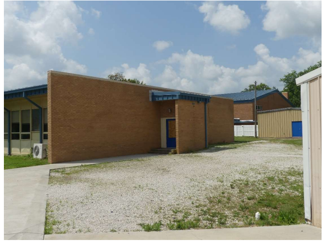
6. North side of the east building section.
