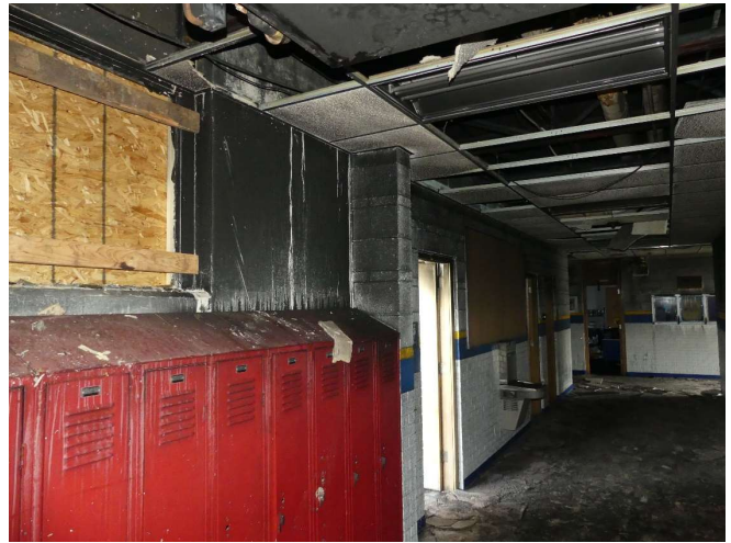
16. Looking east along the east-west hallway.
