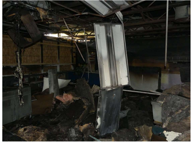
22. View into the west classroom in the east-west oriented building segment.
