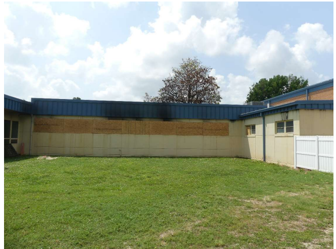
8. North side of the center building section.
