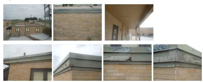
BRICK WALLS: The majority of the building is constructed with Blond Brick that has a 'vertical scratch' finish instead of a smooth finish. The condition at most of the brick and mortar is good, with few cracks or loose mortar. The masonry should continue to protect the building for many decades to come. The brick could use a good low pressure spray wash and scrub to remove accumulated grime, stains, mold and mildew.
