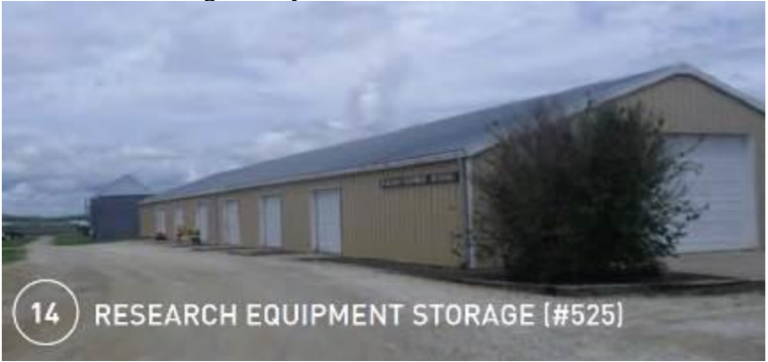
Existing Research Equipment Storage Building
